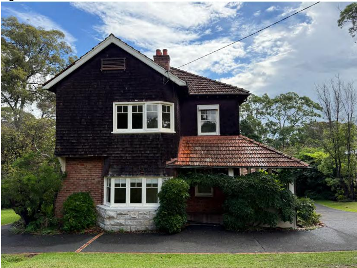
Figure 1: View of front elevation
