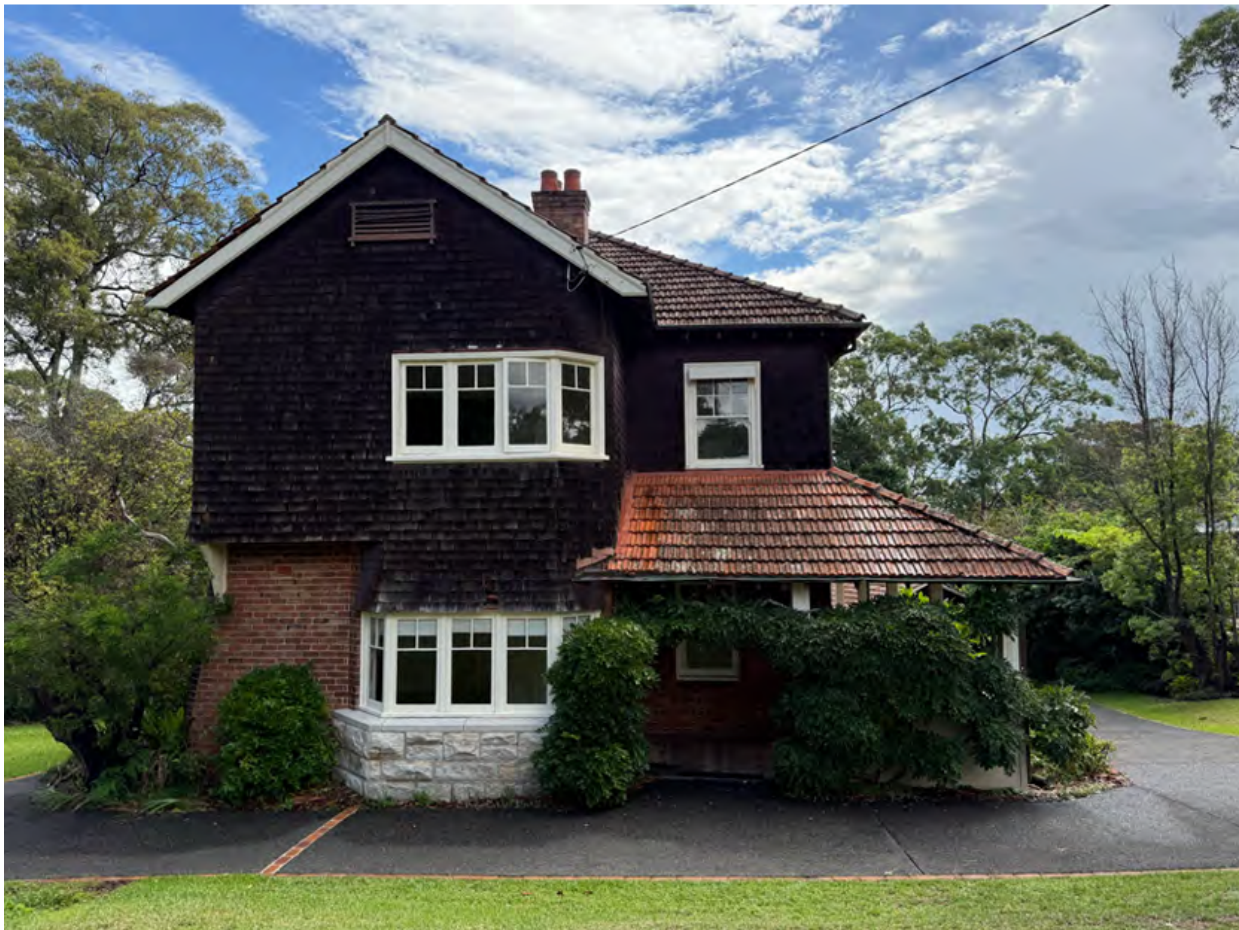
Figure 1: View of front elevation
